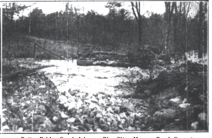
Potter Bridge Carried Away—Rice City—Moosup Road, Coventry
